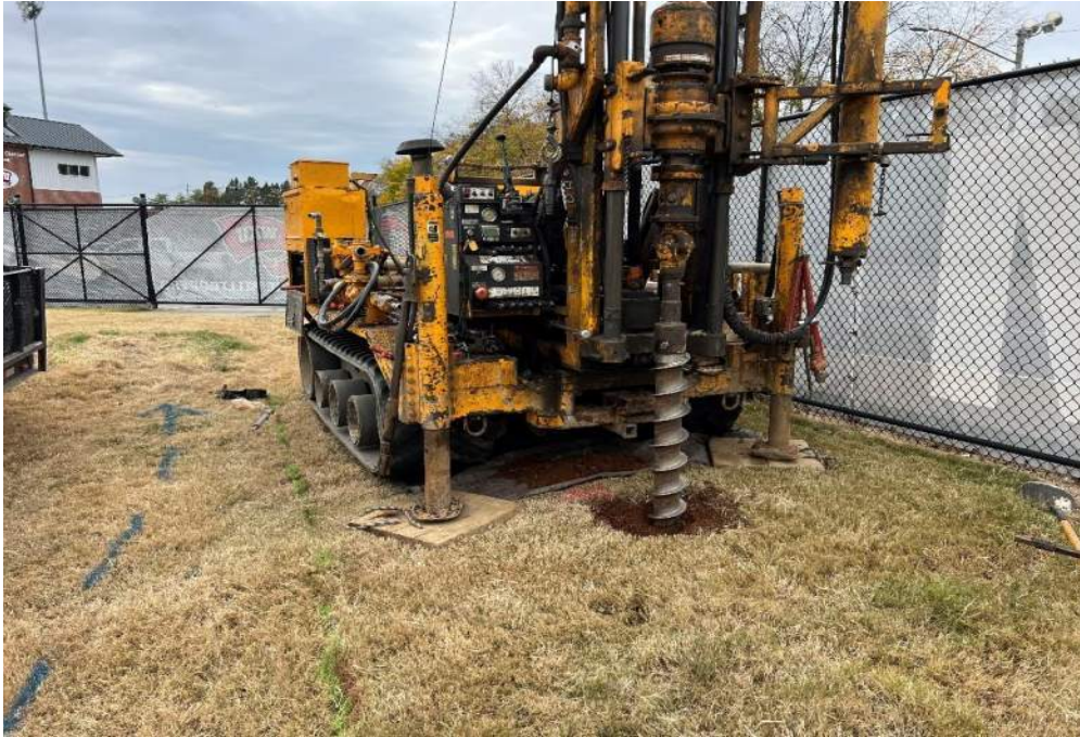
PHOTOGRAPH 9 - DRILLING SOIL TESTING BORING B-12
