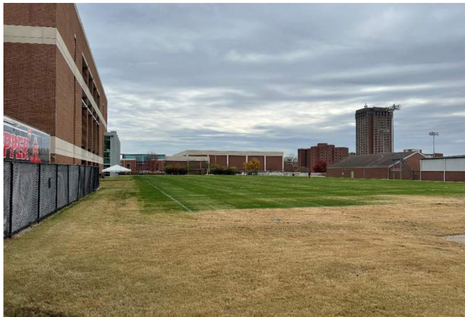
PHOTOGRAPH 2 - VIEW OF SITE FROM NORTH TO THE SOUTHEAST
