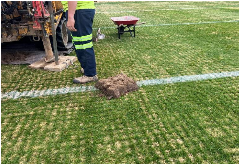
PHOTOGRAPH 8 - PLAYING SURFACE REMOVED PRIOR TO DRILLING
