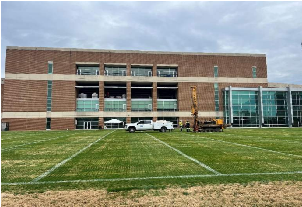
PHOTOGRAPH 7 - SETTING UP ON SOIL TEST BORING B-7
