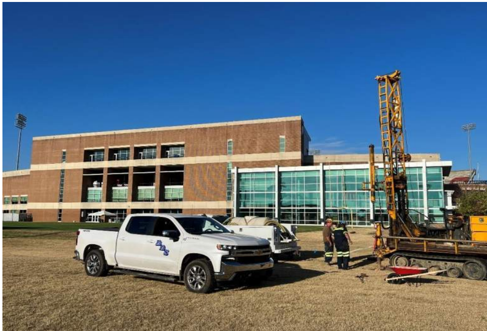
PHOTOGRAPH 10 - SOIL TEST BORING AND ROCK CORING AT B-3
