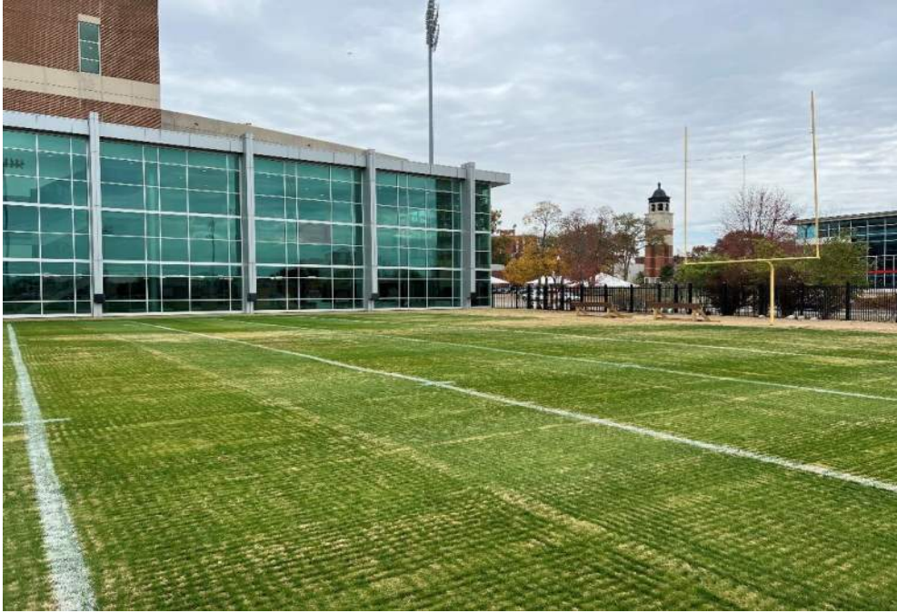
PHOTOGRAPH 5 - VIEW FROM PRACTICE FIELD TO THE EAST
